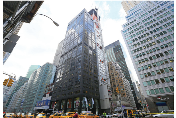
The buyers of a property at Park Avenue and 57th Street are hoping that a taller tower being built next door will add to its value. Credit Ruby Washington/The New York Times
